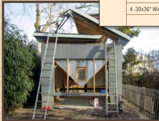
Jacking up Roof
