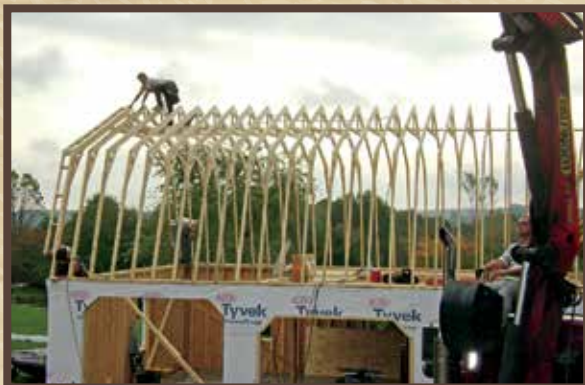
Build On Site
