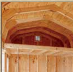
4' Deep Loft in Dutch Barn
