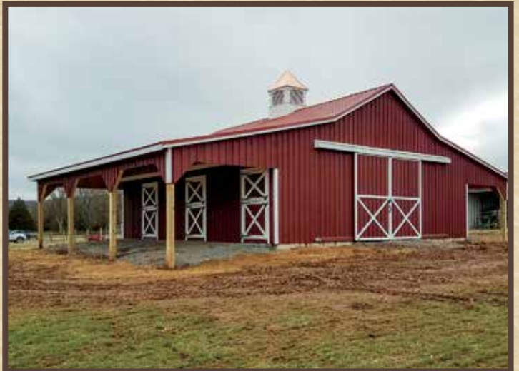
(523) On-Site Build Horse Barn
