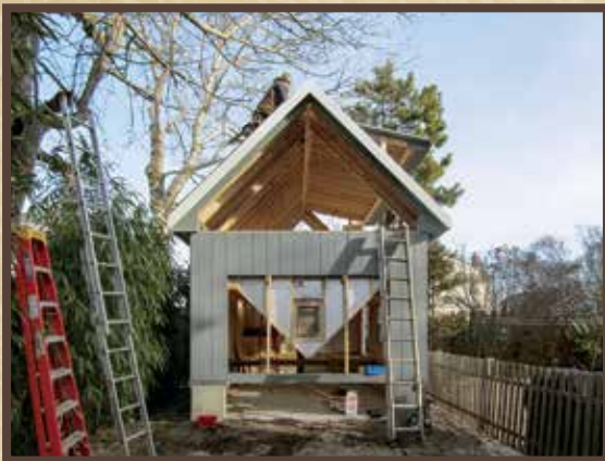
Hinge Roof Under Construction
