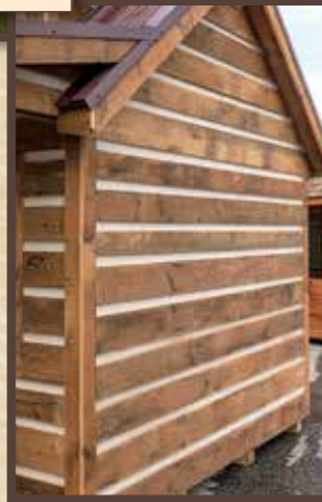
Old Reclaimed Siding with Chinking
